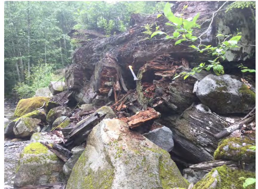
Right Bank Abutment when facing downstream
