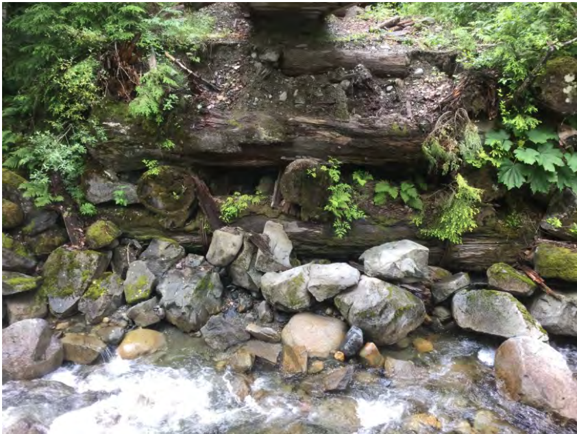
Left Bank Abutment when facing downstream
